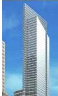
The new Goldman Sachs building at West & Vesey: not available to mere mortals
